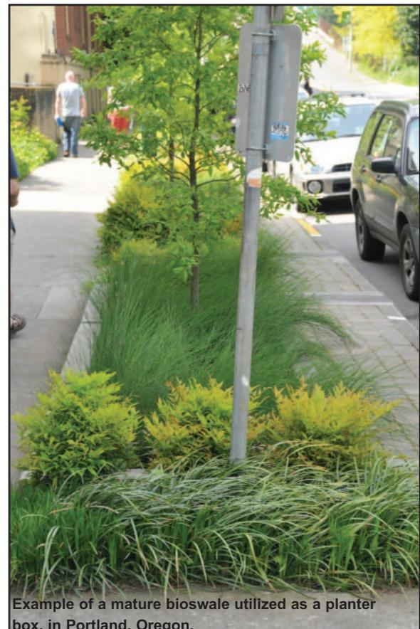
runoff is managed onsite instead of direct conveyance through the storm sewer system; therefore, the peak runoff events should be reduced by some margin. Runoff will be allowed to infiltrate thereby recharging the groundwater table. The bioswales can also reduce sediment and nutrient runoff.
